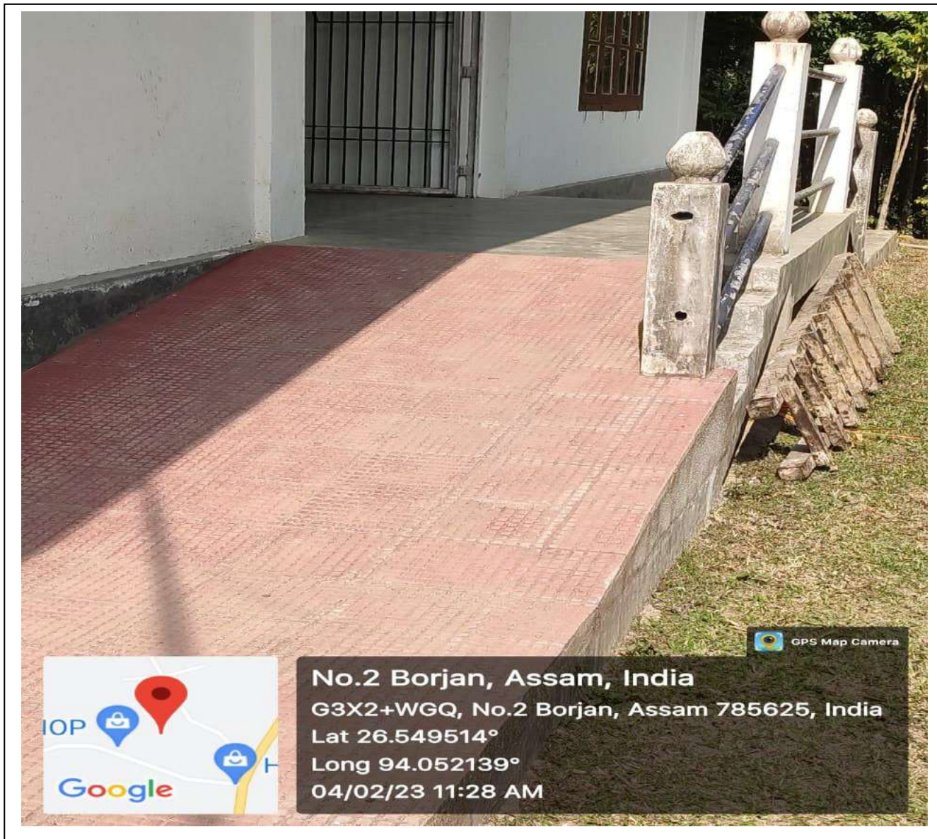
Ramp in front of Classroom and Library Building
